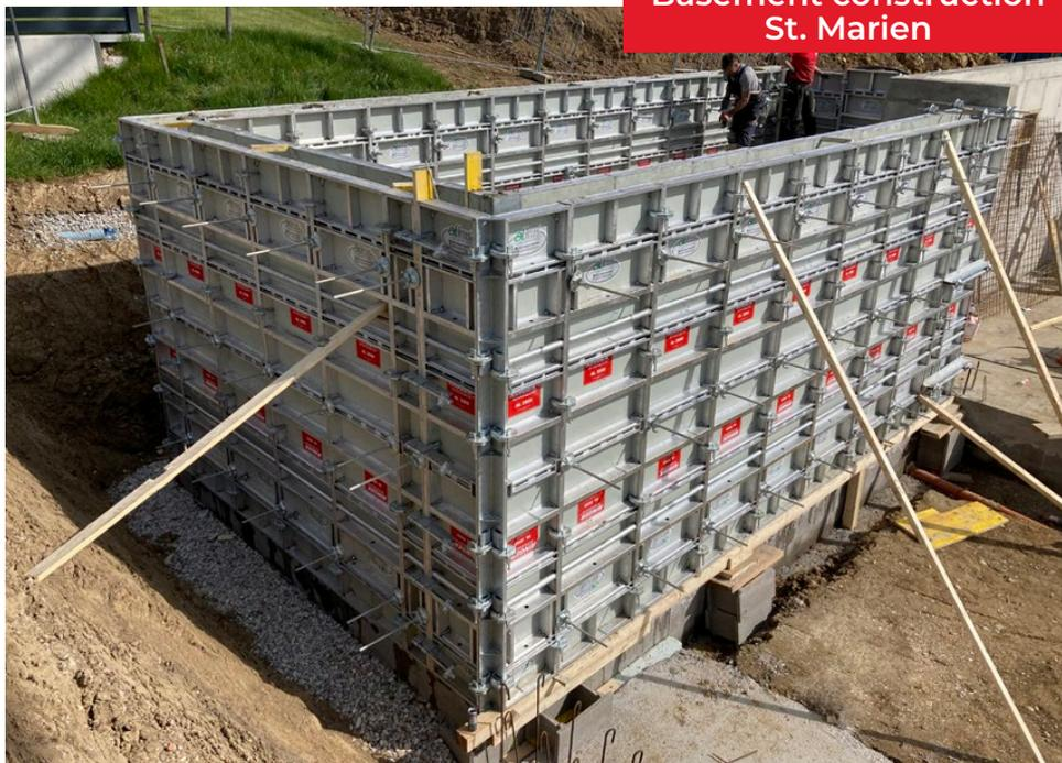
System 2000 with 3m panel height and Alkus solid plastic plywood.
