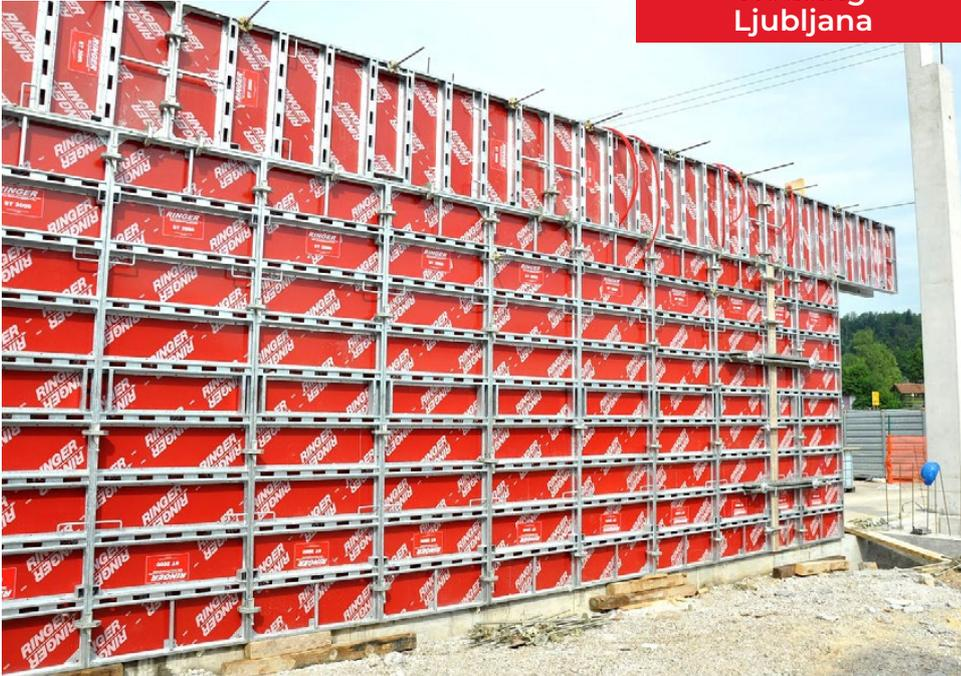
The ST2000 panels can be used vertically or horizontally, as required.
