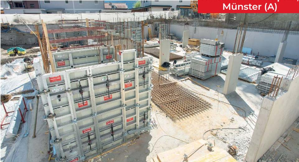
Thanks to the tie rod storage space, the tie rods are always where they should be.
