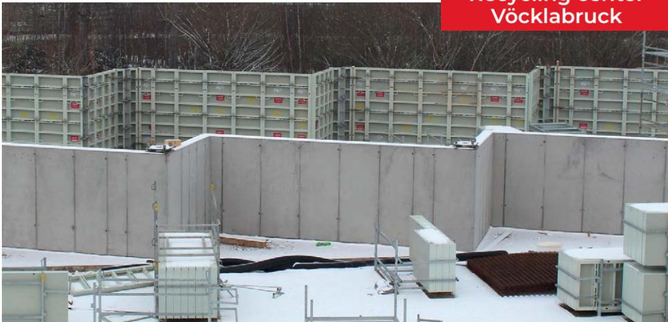
The retaining wall was formed using Alu Master panels with Alkus plywood
